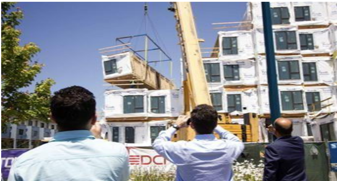
Crane Installation of Volumetric Modular Units (On-Site Assembly)[19]
